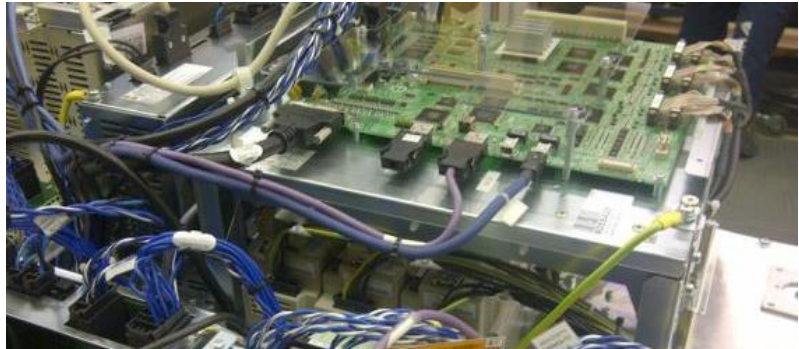
Controller & Cabinet Assembly in Torsas, Sweden
